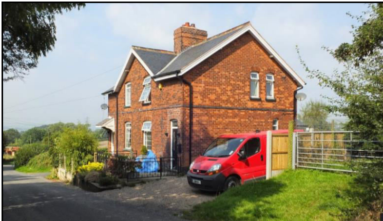
Calow Green gatekeeper's cottage looking west. The gated level crossing was on the far side of the cottage. photo: "Ian T"/Google Earth
